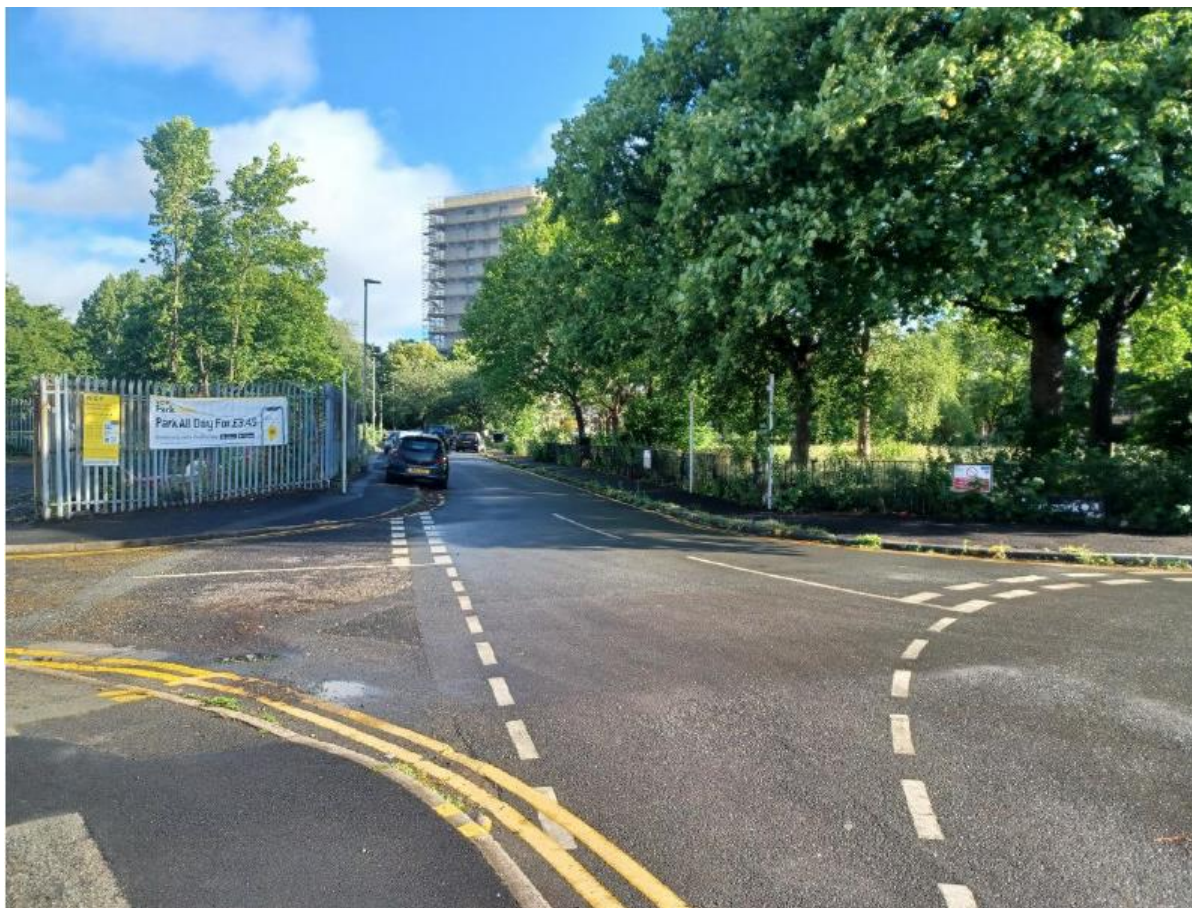
Photograph of the site at the junction of Jersey Street and Wadeford Close
